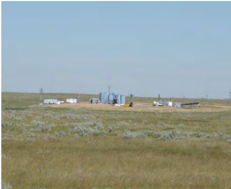
Picture 1. Battery station in the Manyberries oilfield.
