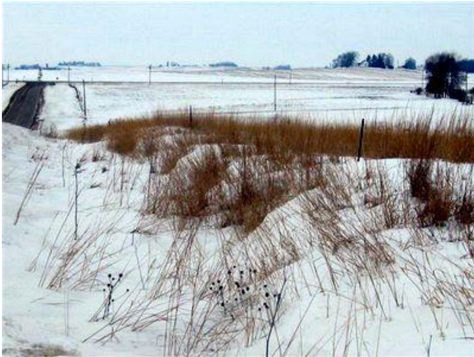
Fig. 11. Integrated roadside vegetation management at work: Using tall native grasses and wildflowers on the backslope keeps snow off a county road in Iowa. Shorter native grasses are planted along the shoulder to eliminate the need for mowing, while wet meadow species in the ditch slow down runoff and enhance water infiltration. Photo courtesy of Iowa Department of Transportation
